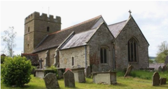
St Swithin's, Clunbury
