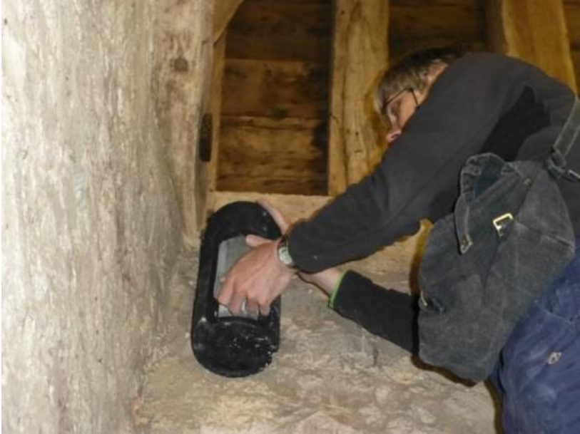
Bat box being installed inside a church tower
