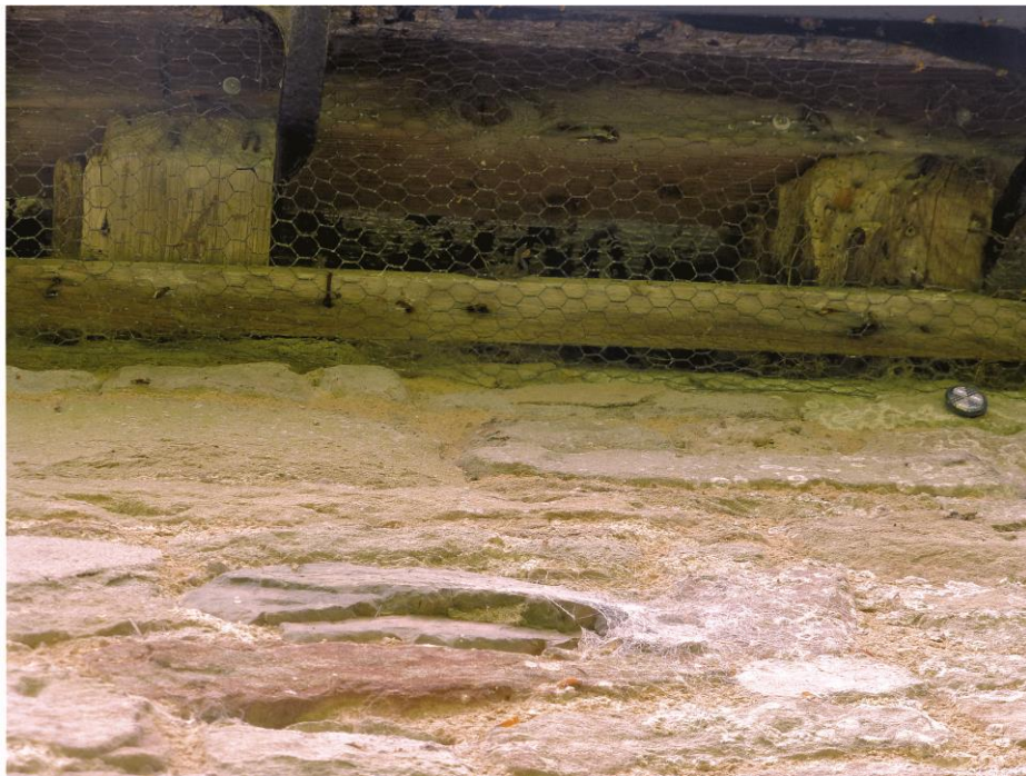
Eaves meshed at a Herefordshire church where swifts were observed locally
