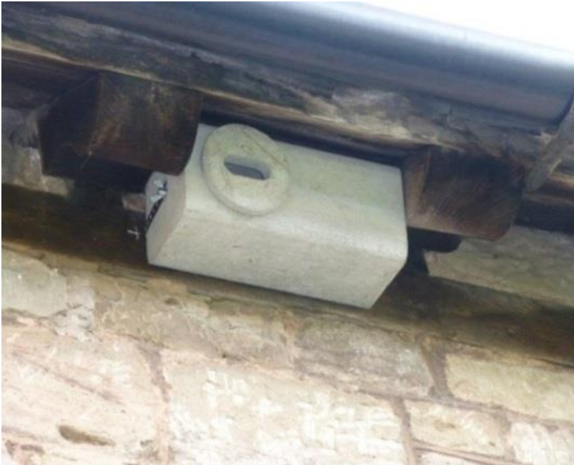
Swift boxes are installed under the eaves
