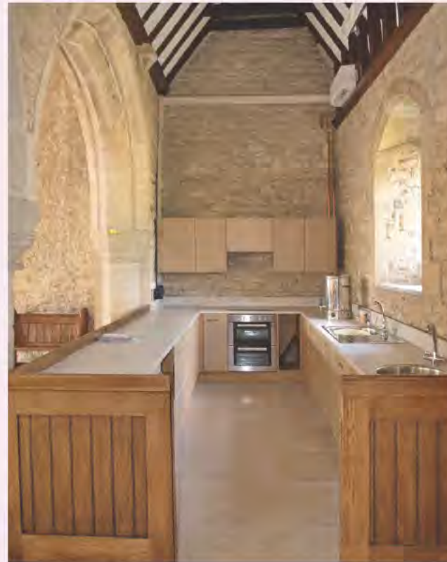
Completed kitchen at Stadhampton © Mike Peckett June 2013
